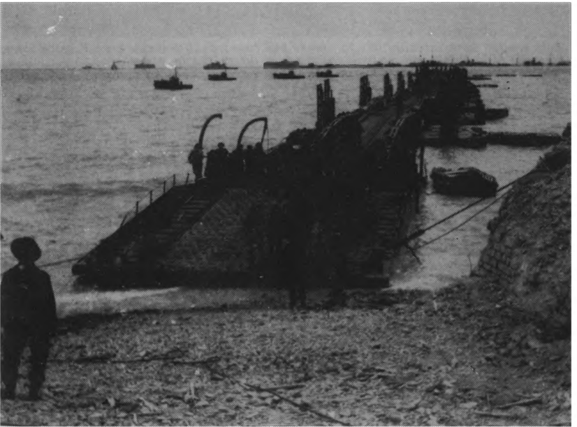
Shore ramp boat and First Portion of roadway drawn up on beach at high tide.
