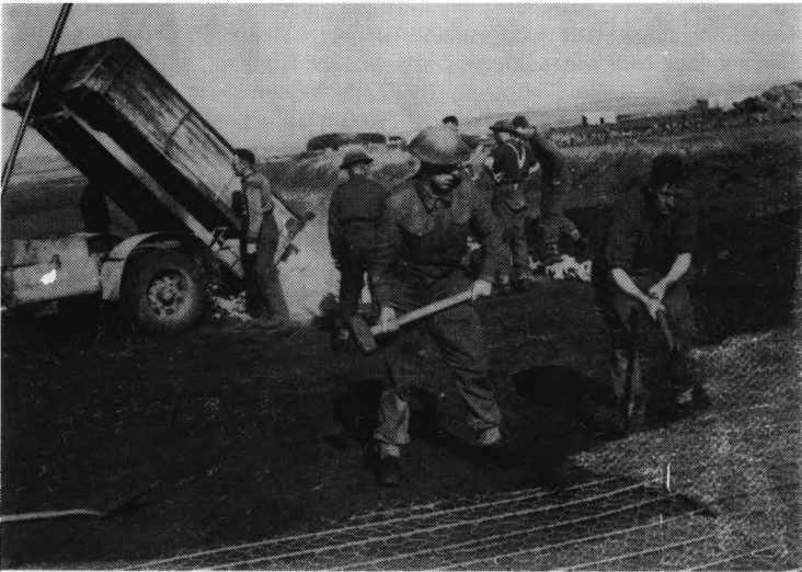
Laying the foundation of the runway and fixing the Sornerfeld track.
